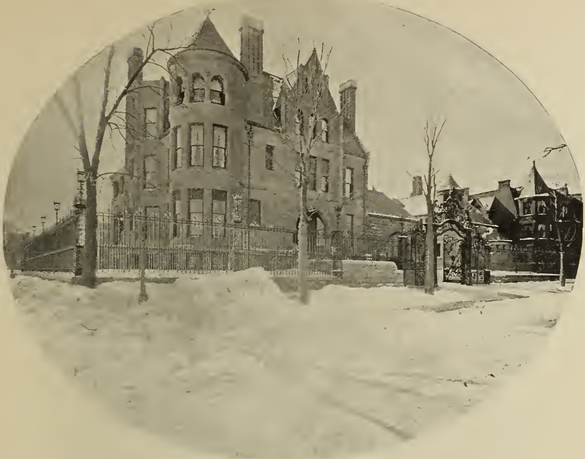
RESIDENCE OF GEN. JOS. T. TORRENCE, LAKE SHORE DRIVE AND BELLEVUE PLACE, CHICAGO—GATEWAY AND FENCE. (See ORNAMENTAL IRON, March, 1894.)
